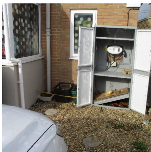
Figure 3: Cabinet built around charger
