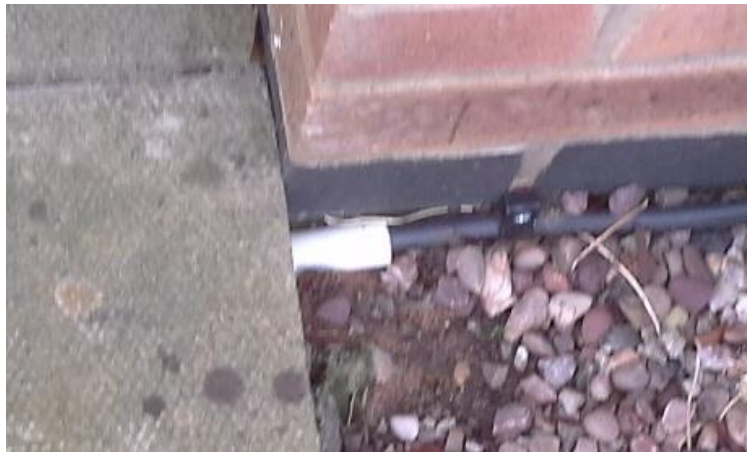
Figure 6: Cable under paving stone
